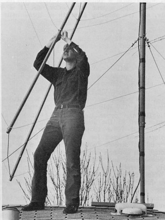
Fig. 5 -- NØART stands on the roof to add 12 polyester cross ties by rotating the quad in the vertical plane. Polyester is strong and stretches very little. It is also highly resistant to sunlight.
