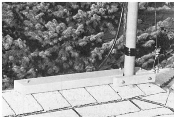
Fig. 10 — A V-cut 2 x 4 and screw-adjustable block make a roof-mounted mast clamp to prevent rotation. The roof was sealed before clamp installation. A heavy ground wire is attached to the mast for lightning protection. Dressed along the mast are coaxial and rotator control cable, which has been wrapped with grounded copper mesh to prevent RF pickup from feeding the shack.
