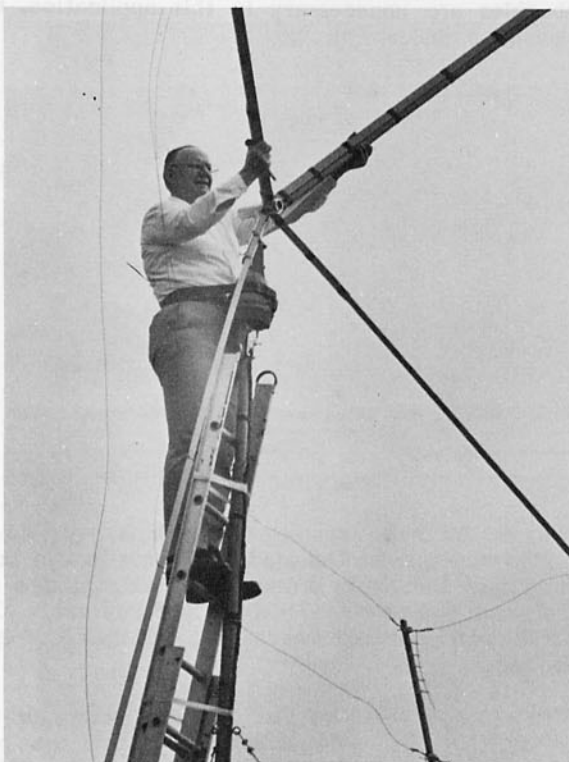
Fig. 4 — NØARQ slips the reflector element onto the mast T. A 63-inch spruce tie bar supports 12-inch x 3-inch mini-stubs in the bottom center of each reflector loop.
